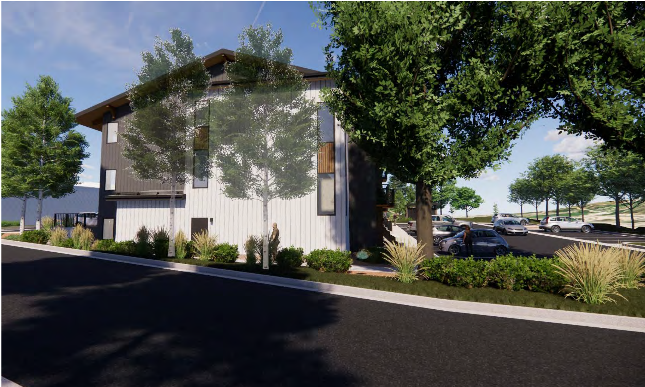
SOUTH FACING VIEW
