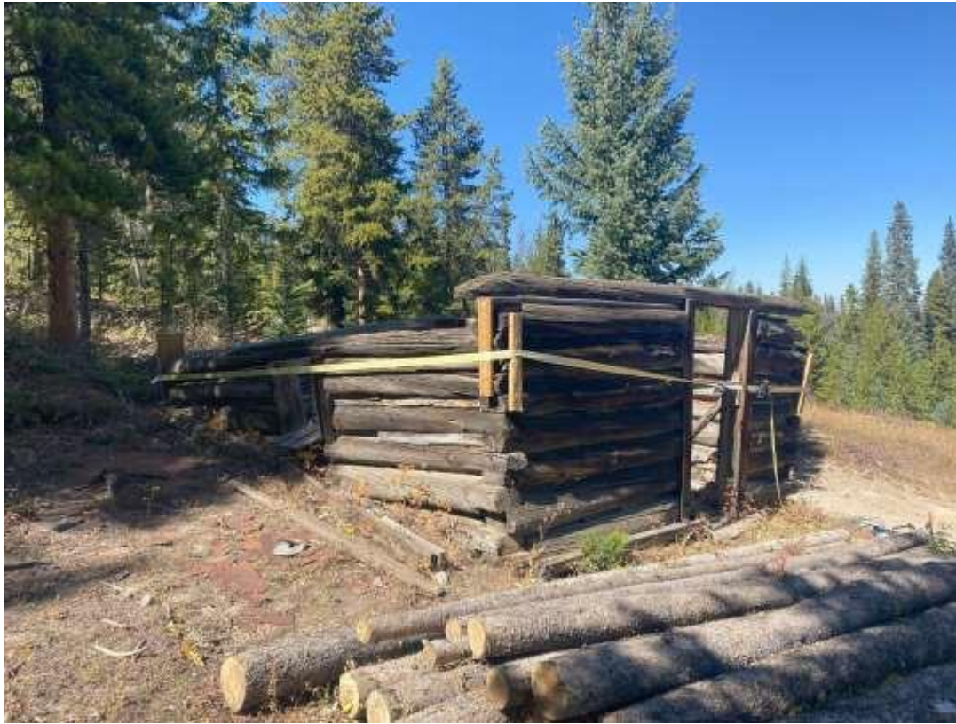
Current photo of Preston cabin 1; logs to be used are in the foreground
