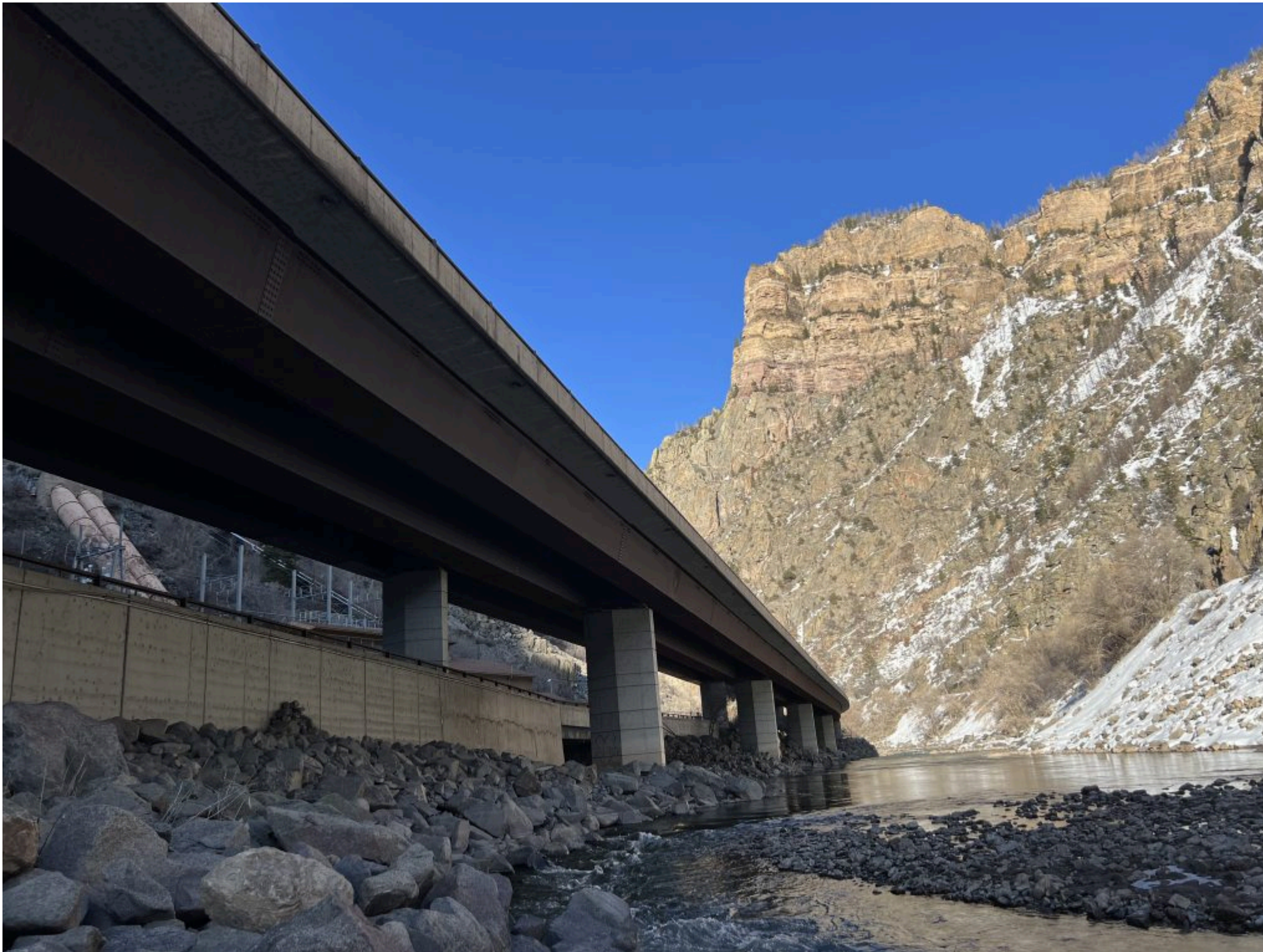
Part of the Shoshone Hydroelectric Plant in Glenwood Canyon is seen from the Colorado River. The Shoshone water rights are a package of two connected water rights, which together are entitled to 1,408 cubic feet per second of water, or 1 million acre-feet of water per year. Zoe Goldstein/Vail Daily
