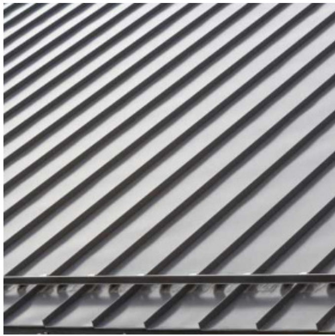
STANDING SEAM METAL ROOF
