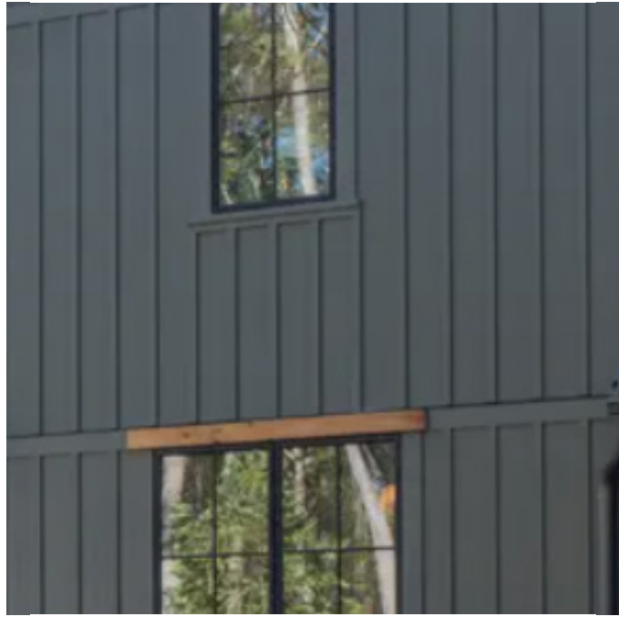
BOARD AND BATTENV CEMENT BOARD
