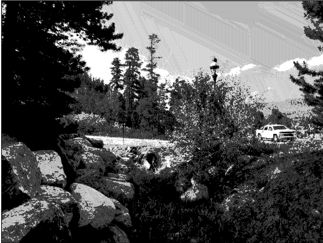
Photo 7 – Looking north at the vegetated (non-wetland) entrance to the culvert under Woods Drive (July 19, 2021)
