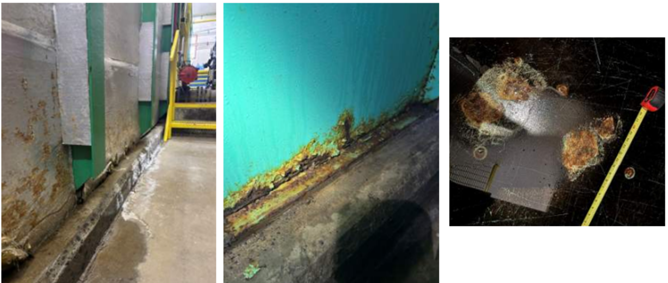
Photos of the steel water treatment plant tanks showing the pitting, corrosion, and leaks in the tanks
