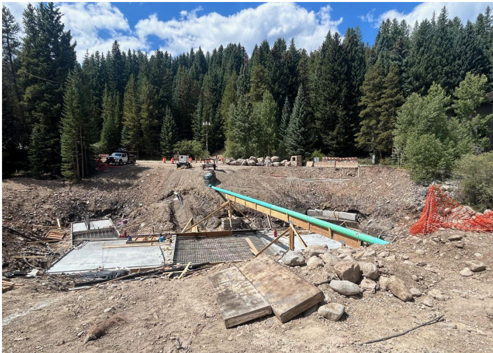
View looking west in the excavation for the new bridge for Broken Lance Drive. The sanitary sewer line was installed and the fir concrete placement for the bridge footers is completed.
