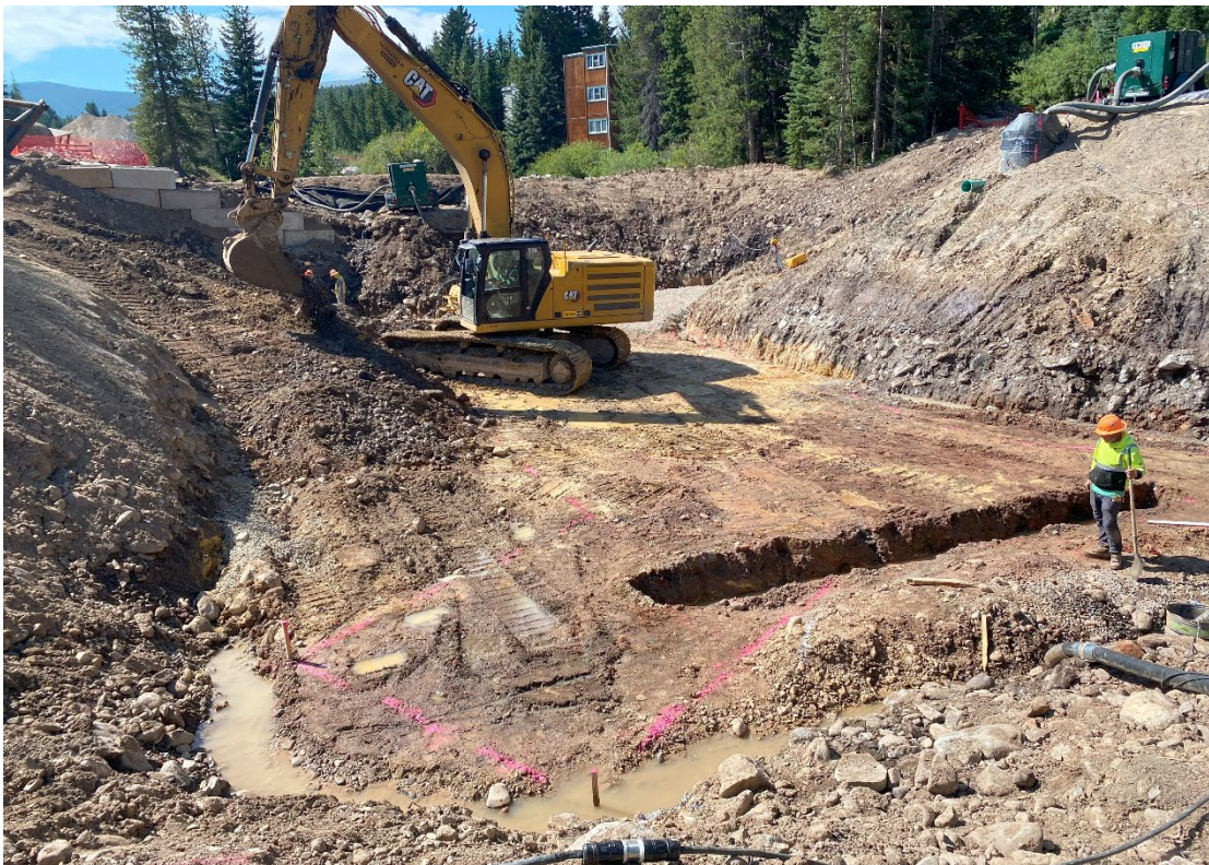
View looking downstream in the excavation for the new bridge for Broken Lance Drive. The Blue River and sanitary sewer are currently being diverted around the excavation.
