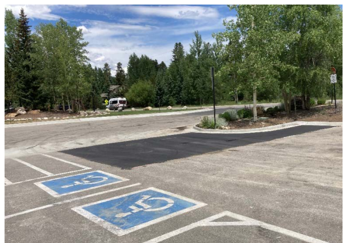
Ice Rink concrete pan and curb and gutter replacement.
