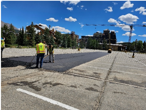
F-Lot patching and pothole repairs.
