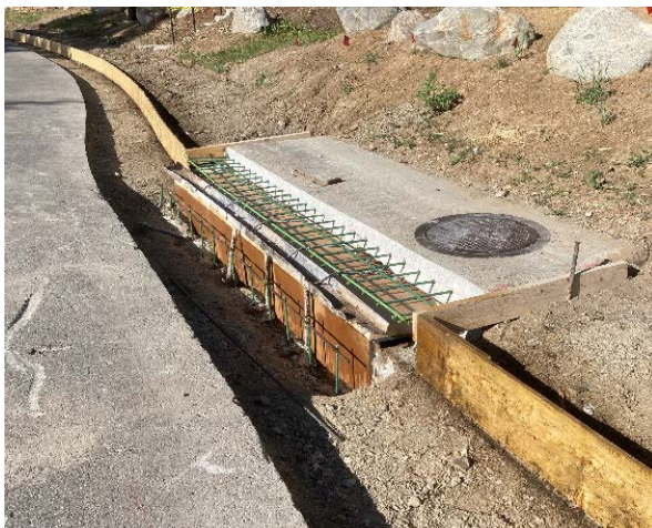
Village Road inlet repair and concrete replacement.
