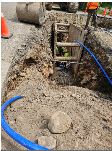
New water main installation at the White Cloud – Broken Lance Intersection.
