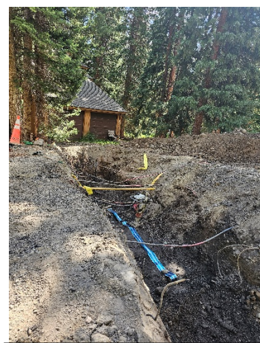
Backfilling a water service connection from the new water main to a home. Multiple utility crossings encountered during service connection.
