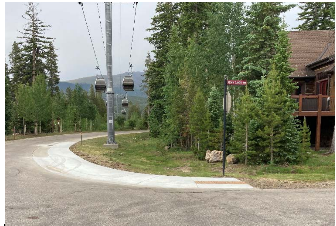
Shock Hill concrete sidewalk and curb ramp replacement.
