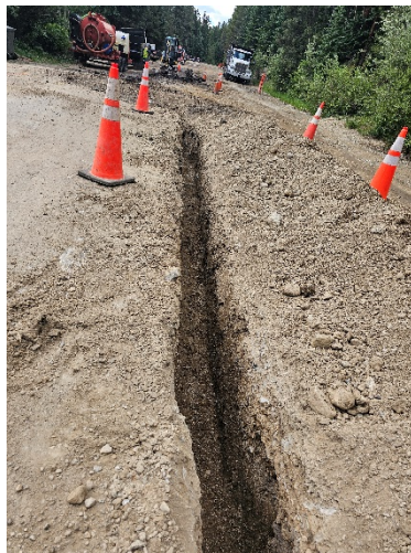
Fiber conduit being installed within the work zone of Broken Lance Dr for future fiber network.
