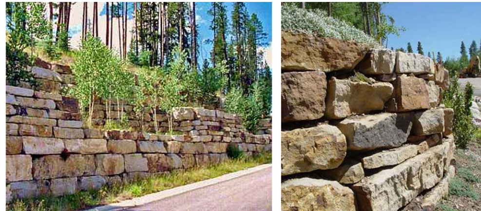
BOULDER WALL COURSING AESTHETIC INTENT, AND SILOAM STONE MATERIAL
