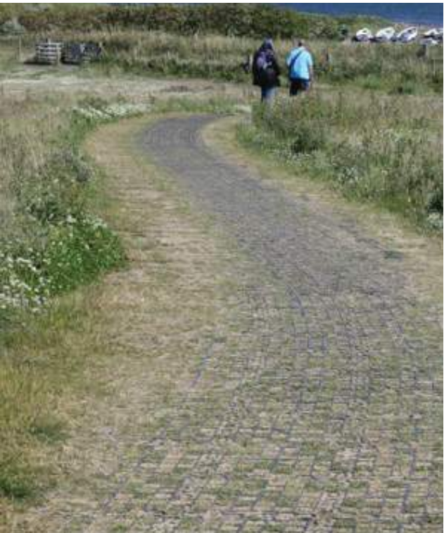
REINFORCED SOFT SURFACE TRAILS
