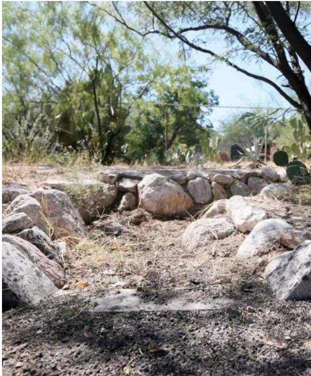
CURB CUT & DRY DRAINAGE CHANNEL
