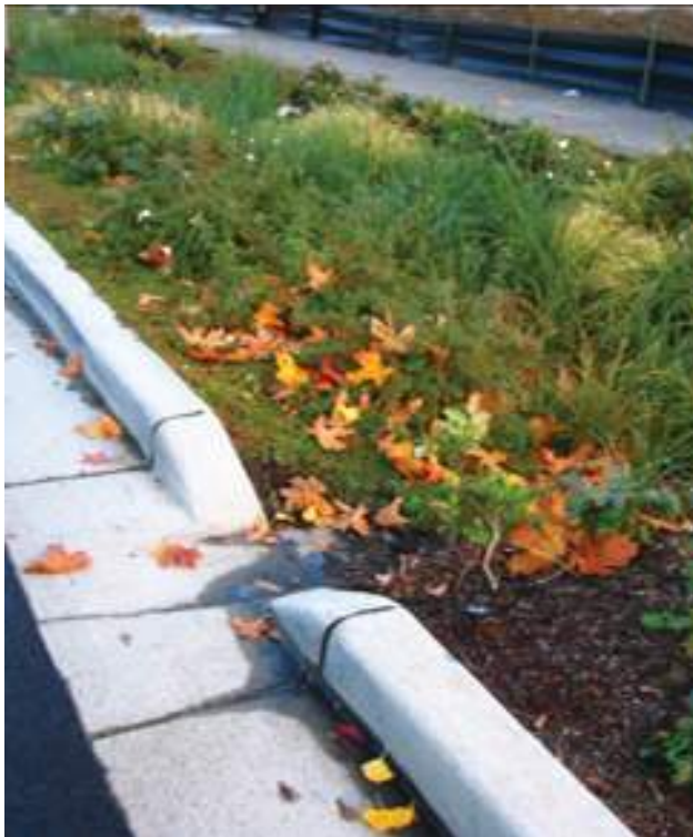
CURB CUT & BIOSWALE
