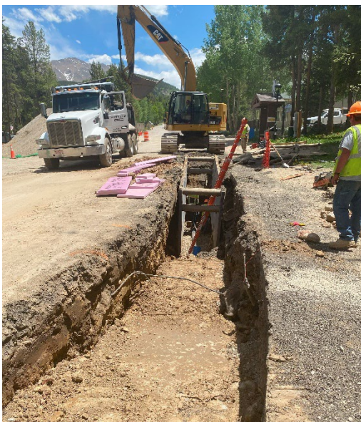
Water line installation utilizing a trench box for safety.
