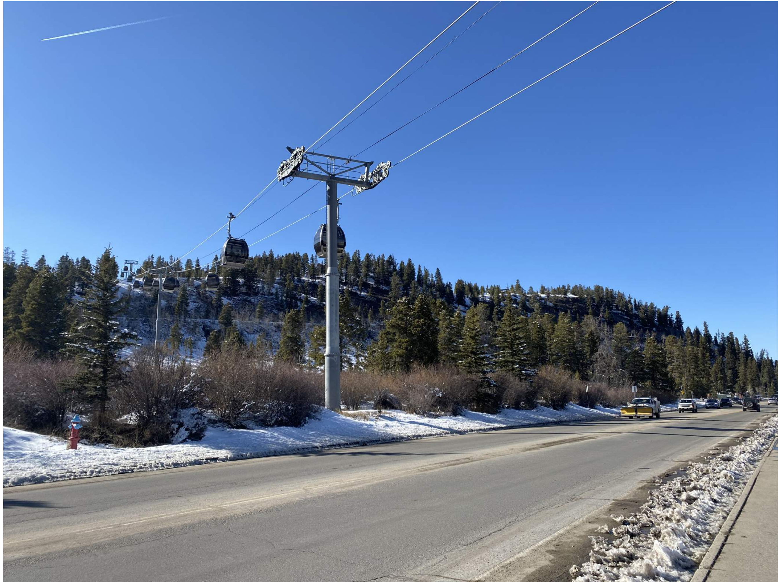
VIEW 3 - NORTH PARK AVE LOOKING WEST
