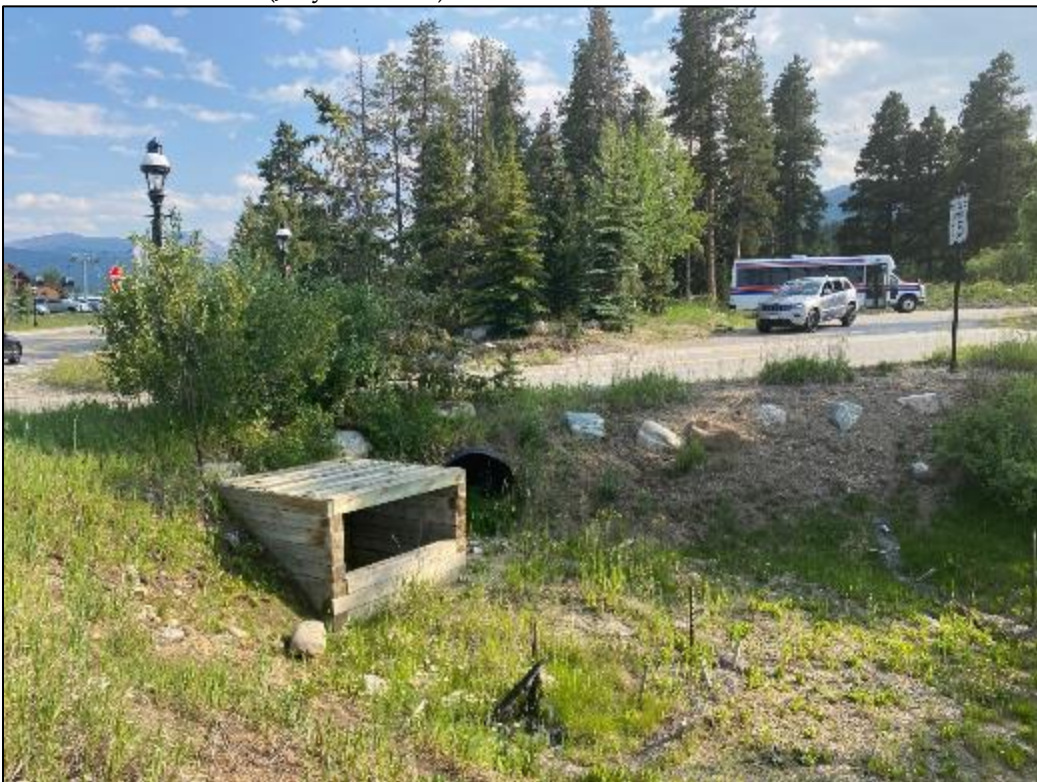
Photo 8 — Looking south at the culvert (black plastic) outlet under Woods Drive, with wooden outlet box to the stormwater system (July 19, 2021)
