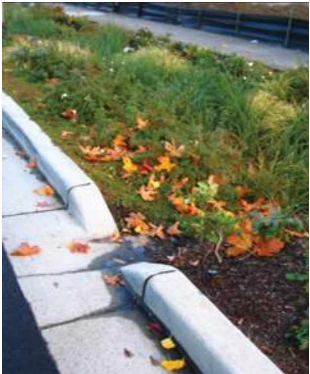
CURB CUT & BIOSWALE
