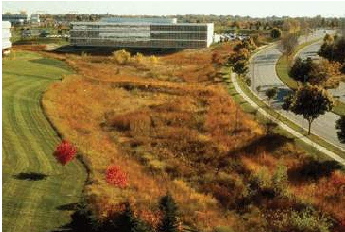
LARGE BIOSWALE MADE UP OF NATIVE PLANT MATERIAL
