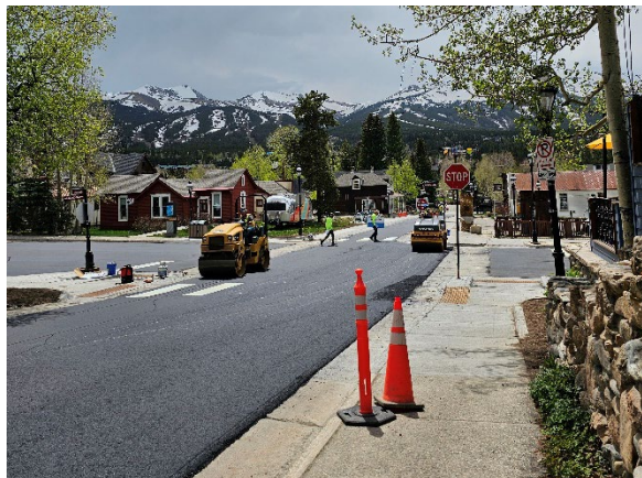
Washington Ave. and Ridge St. intersection paving and ADA curb ramp replacement.
