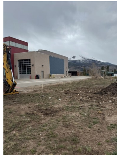
Staking Stormwater Line
