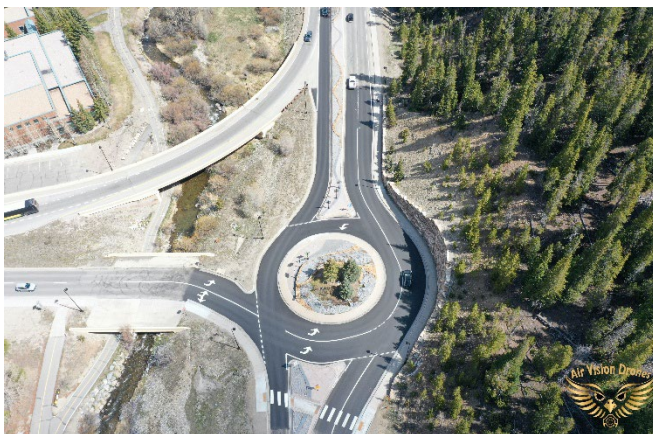
Drone image of the completed paving and concrete repair and replacement of the N. Park Ave. Roundabout.
