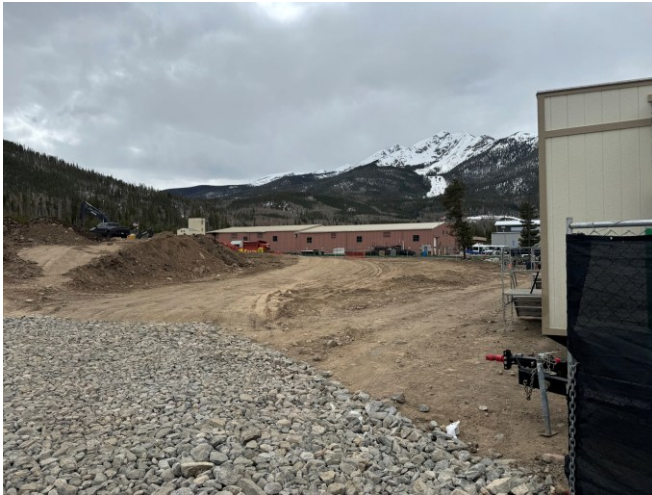
Entrance into Project Site
