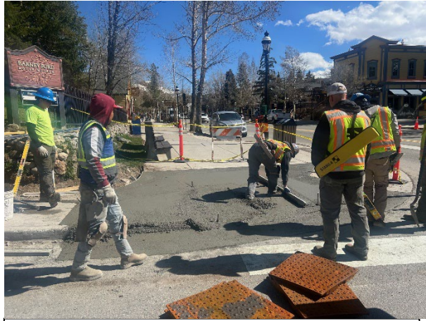
Photos of ADA improvements on the curb ramp located at Washington Ave and Main Street.
