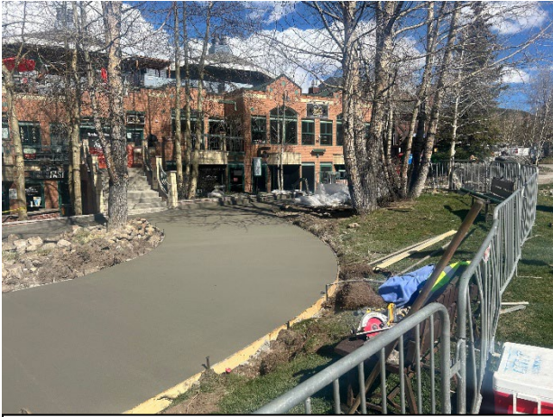
Concrete sidewalk replacement adjacent to La Cima mall.
