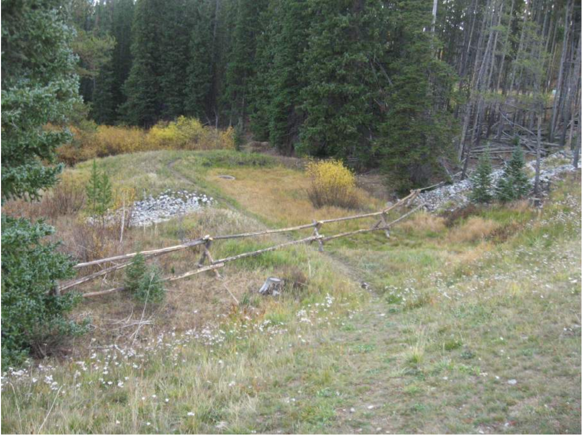
Old detention pond to the southeast of the Peak 8 detention pond.
