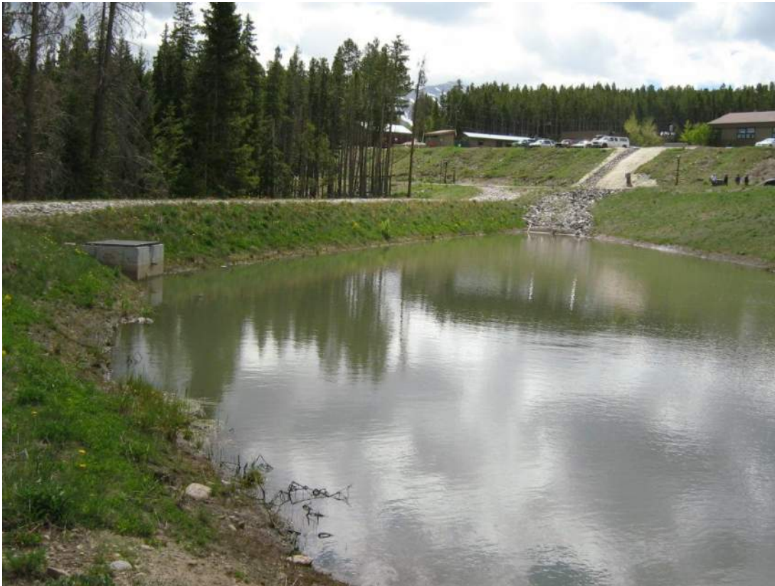
Peak 8 Detention pond. Concrete V-notch outlet is in foreground and riprap drainage swale in the background.
