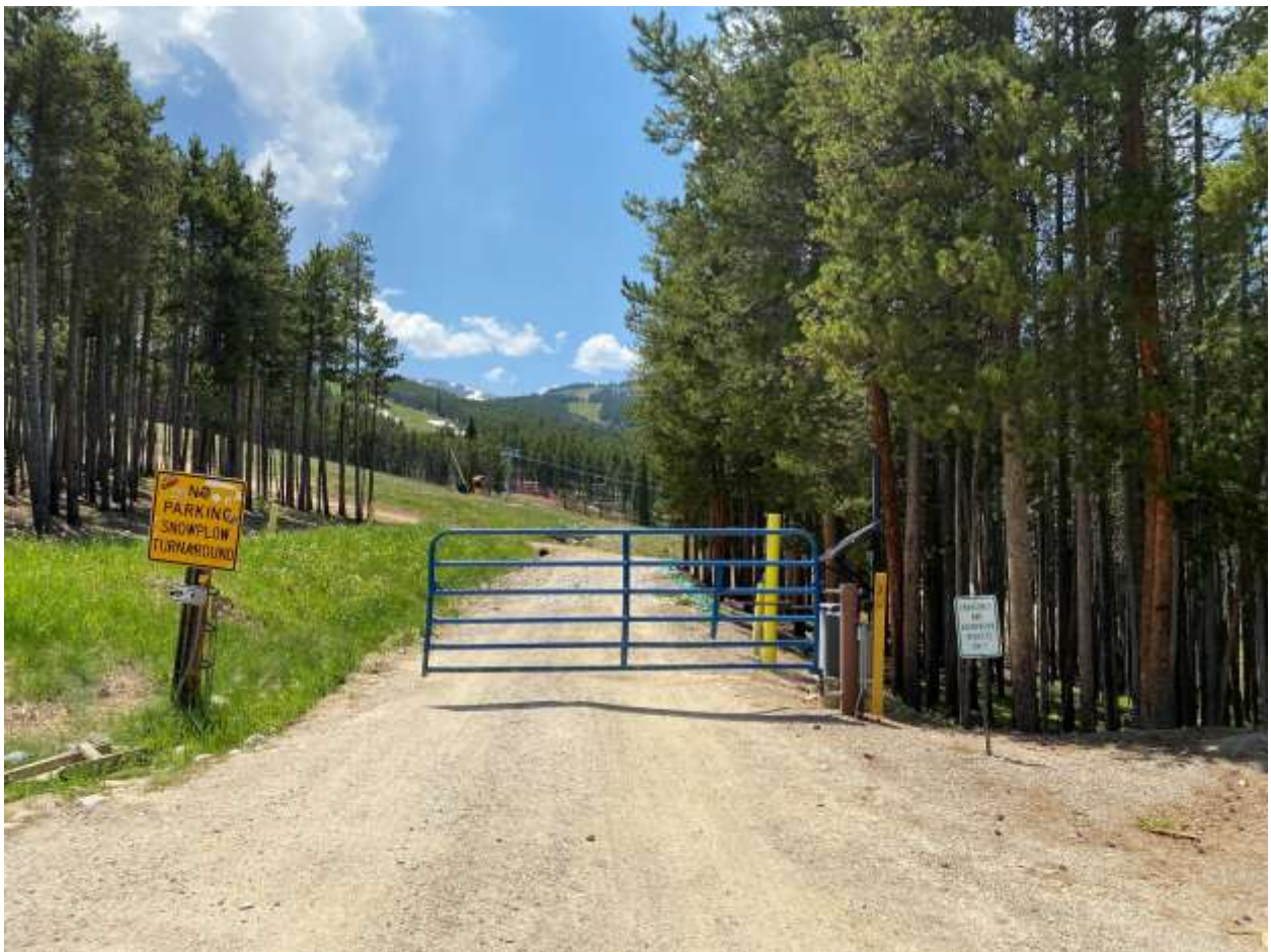
In cul-de-sac looking west.
