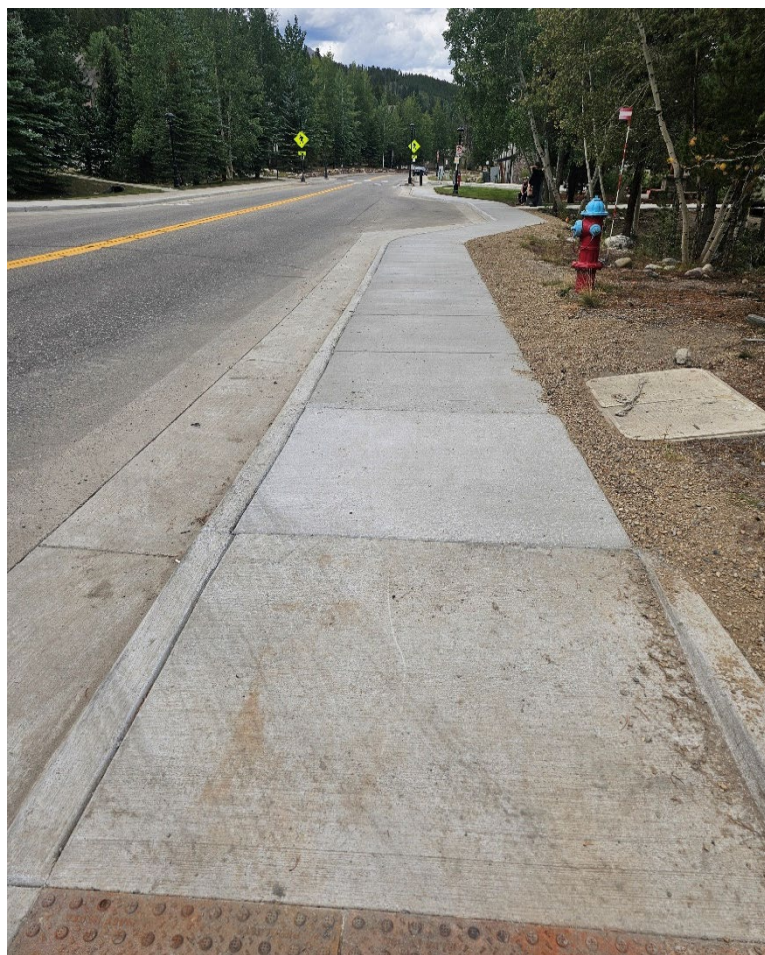
Replaced damaged concrete and made ADA improvements at the Bus Stops on Airport Road near Rankin Avenue.
