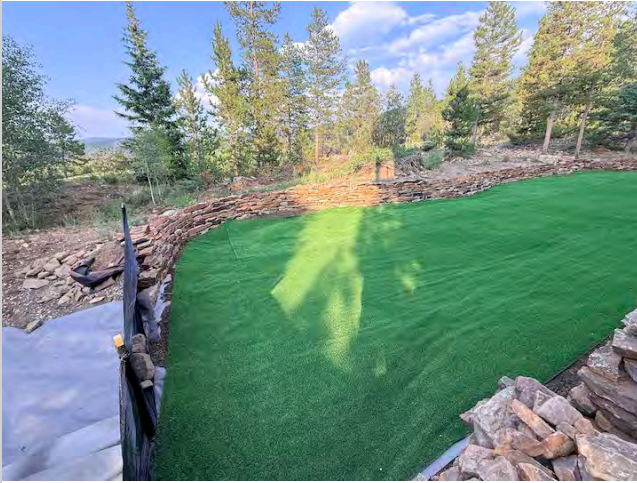
Photo 1: Rear retaining wall overview from the northern side of the residence.
