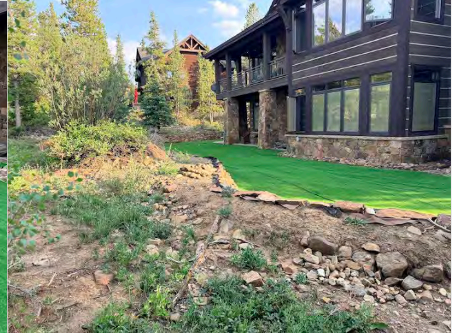
Photo 3: Retaining wall viewed from rear yard closer to golf course safety zone.
