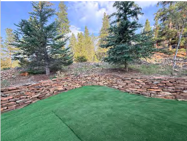
Photo 4: Southern portions of the retaining wall.
