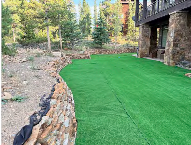
Photo 2: Rear retaining wall overview looking South.
