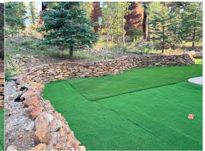
Photo 9: Southern most portion of the wall, connecting over to stairs on the south side of the residence.
