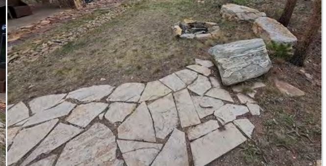
Photo 3: Patio and firepit very uneven and unsafe
