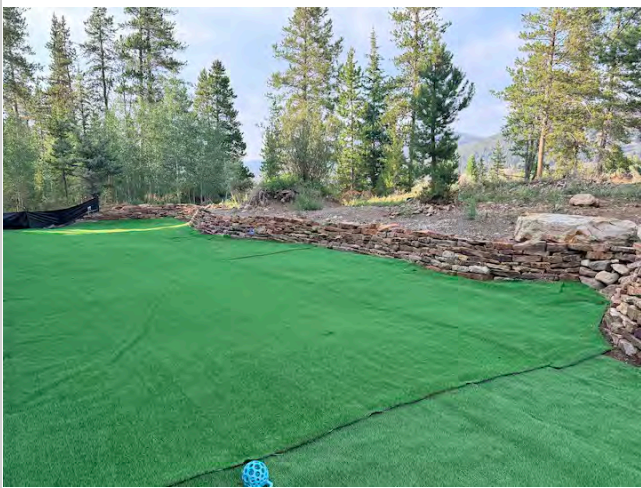
Photo 7: Broad view retaining wall looking North. Portions of the wall on the right side of the paragraph are the "rebuilt retaining wall".
