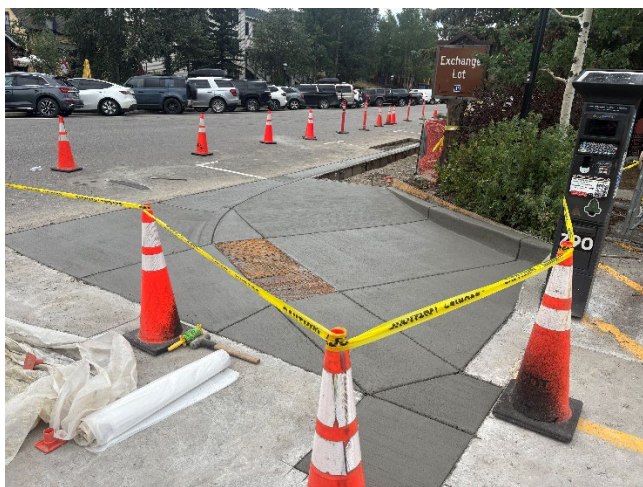
ADA ramp replacement completed at the Exchange Lot along Ridge Street.
