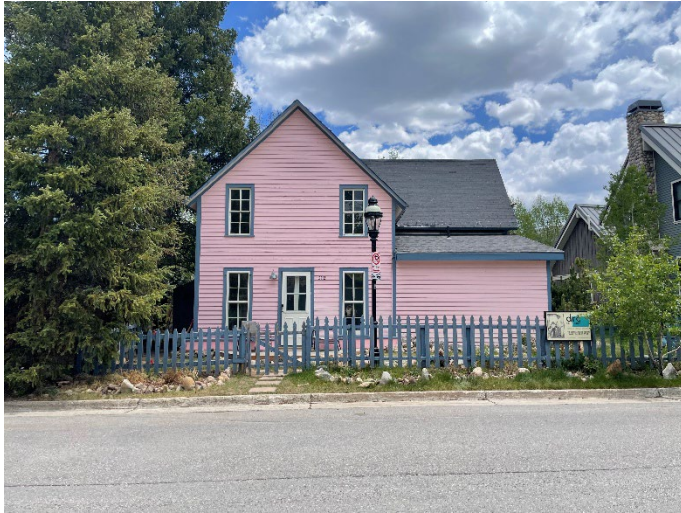
Existing front (west) façade.
