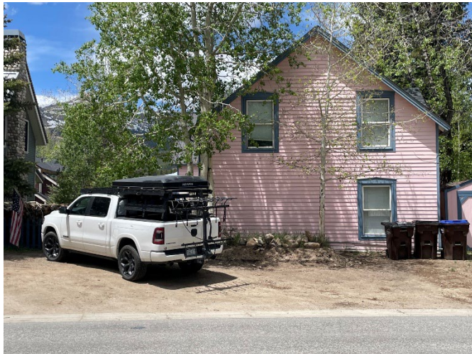
Rear parking within French Street right-of-way
