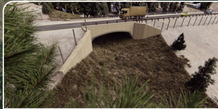
MP 193.0 - Arch Underpass
