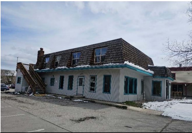
Schoonover building prior to deconstruction in 2024
