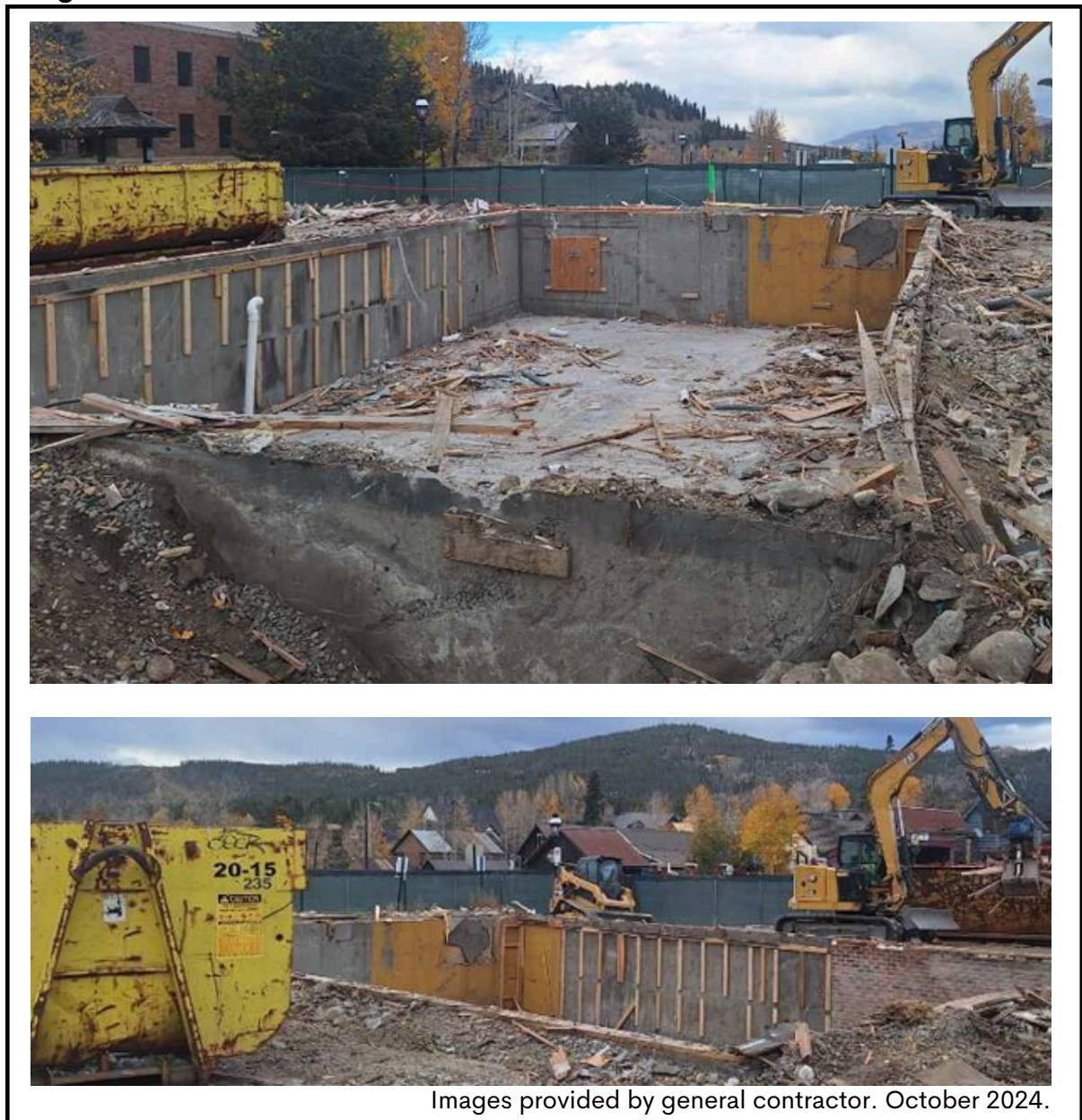
Image 11: Site Concrete Demolition Work
