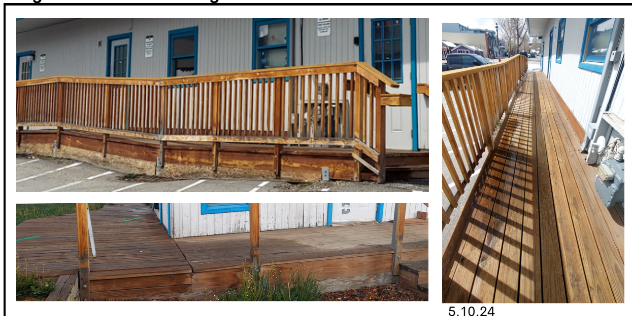
Image 18: Outdoor Decking East and South Side Pre-Deconstruction
