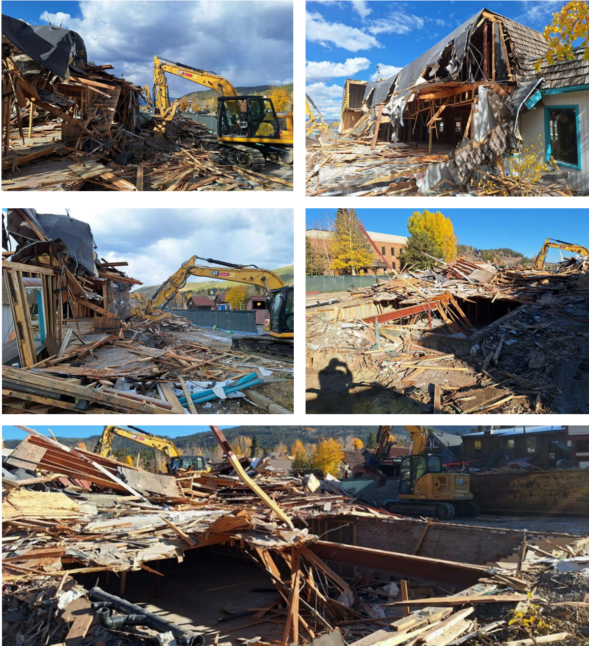
Image 9: Schoonover Exterior Demolition
