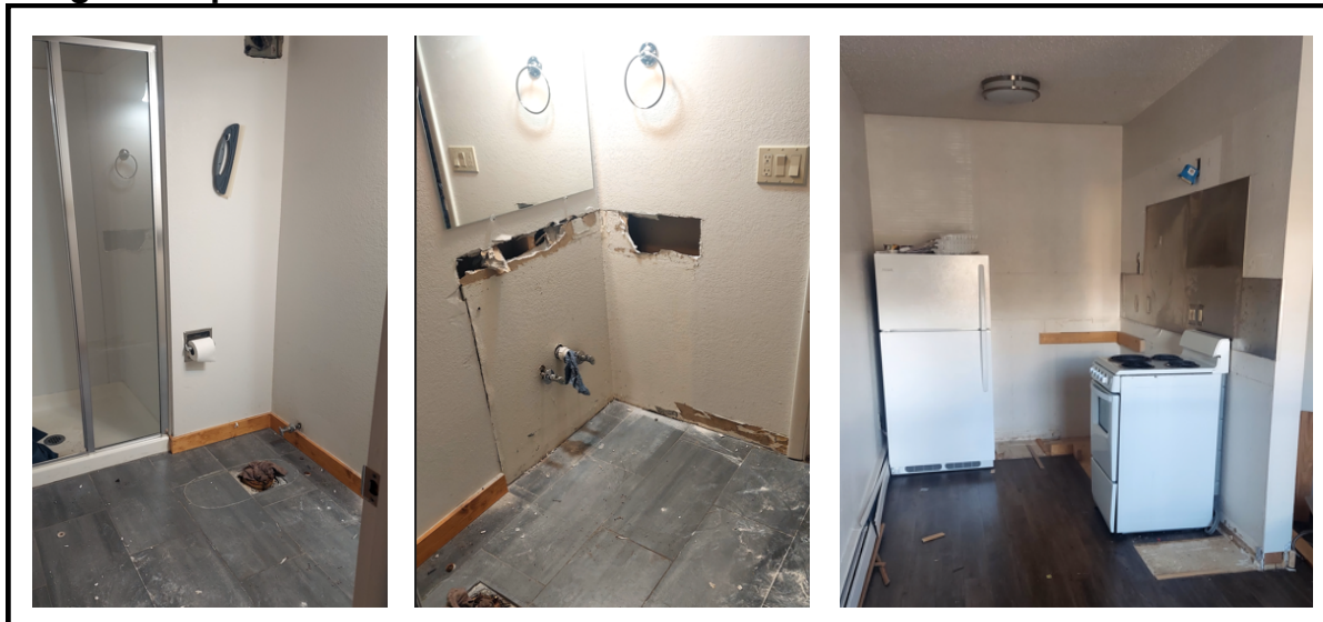
Image 25: Apartment 1 Interior Post-Demolition
