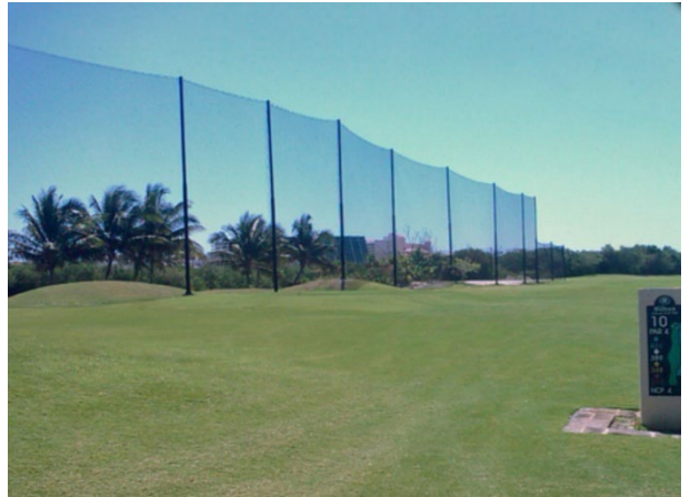
Example photo of a 40' tall netting system
