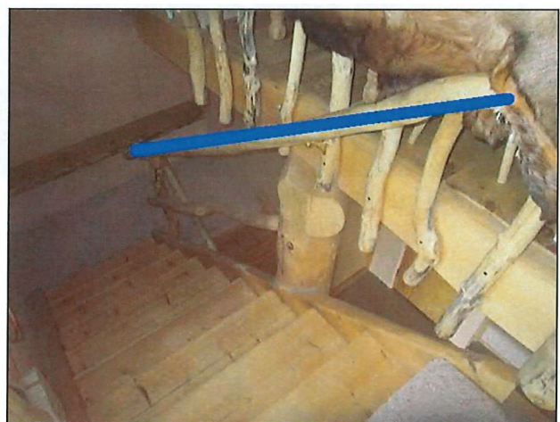
5.4 Install grippable handrail.
