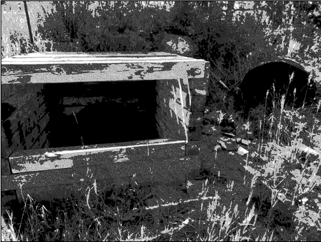
Photo 9 – Close up view of the outlet box showing no signs of flow, looking south (July 20, 2021)
