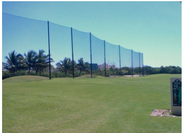
Example photo of a 40' tall netting system
