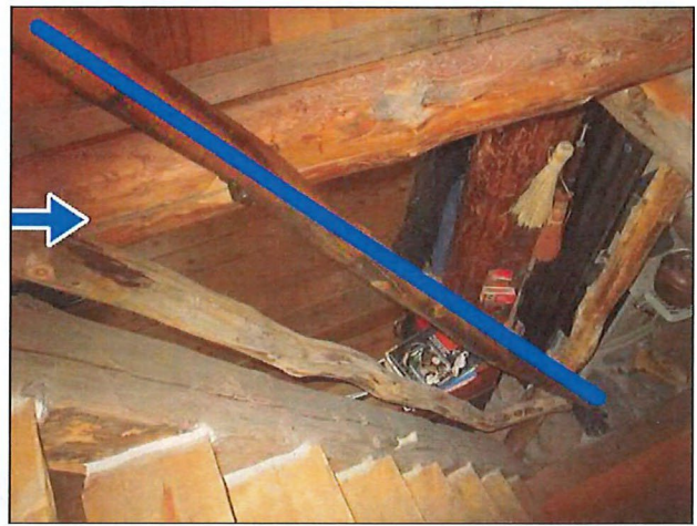
12.3 Rail spacing and install grippable handrail.
